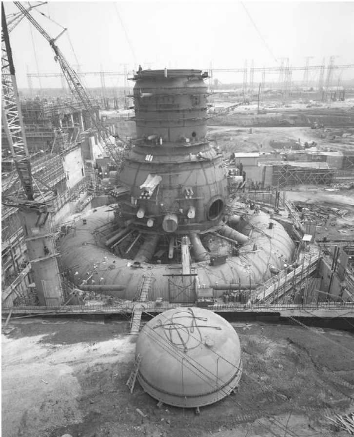
Mark I type PCV under construction in USA. Removed vessel head is downpart of this photo.
